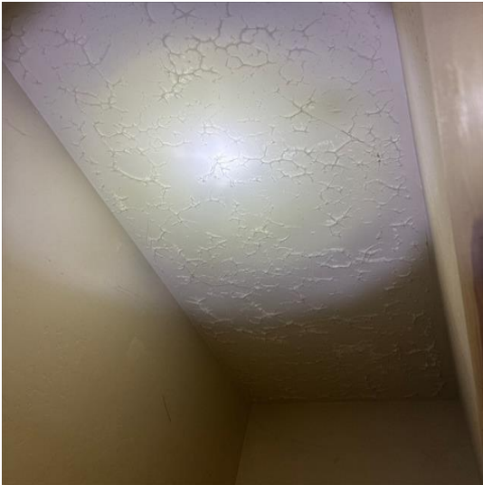
Image Number: 14 Observation: Observation: Bedroom closet overview. Moisture intrusion was NOT reported or observed.
