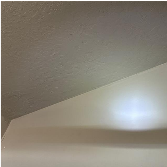
Image Number: 12 Observation: Bubbling paint and moisture staining were observed, indicating active or prior moisture intrusion from above.
