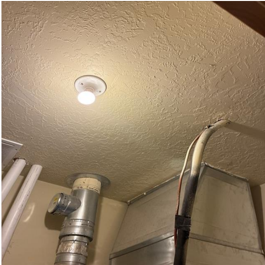
Image Number: 22 Observation: Overview: Moisture intrusion resulting from a roof leak was NOT reported or observed in this room.
